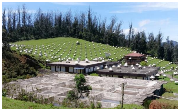
Figure 6. A view of the present-day GRAPES-3 experimental site. The new muon station is located nearby in a single hall. The old muon stations, situated a bit farther away in four different halls, use the similar KGF counters built more than a quarter-century ago.
