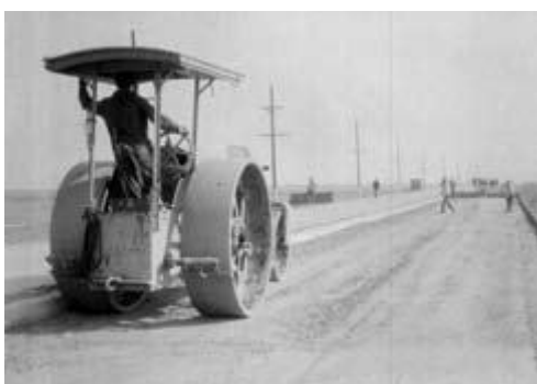
Figure 3a - 1930s: A form of RCC paving is performed in Sweden
