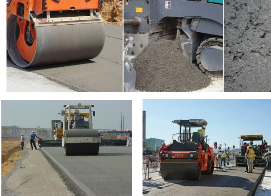
Figure 1 - Construction of a road made of RCC
