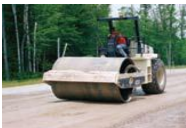
Figure 3b - 1970s: RCC pavements become common for log-sorting yards in Canada
